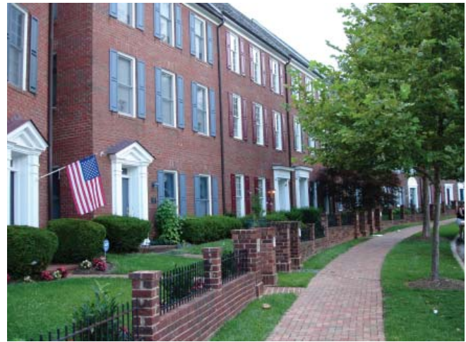
LOW WALLS MAINTAIN PRIVACY GOALS
