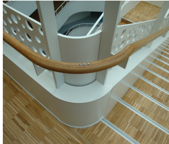
Figure 5. Indicator on handrail is used to identify the location of a stairway.
